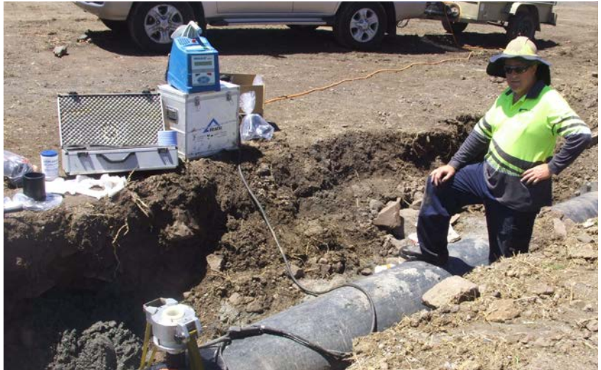
FRIALEN XL 560mm coupler installed near Weeroona Street, Rye - Victoria
