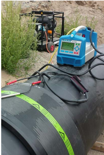
FRIALEN XL 560mm coupler installed near Weeroona Street, Rye - Victoria
